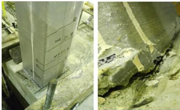
Fig. 10. The cracks of C2G2 column at failure under the lateral load. Separation of the fiber is noticed
