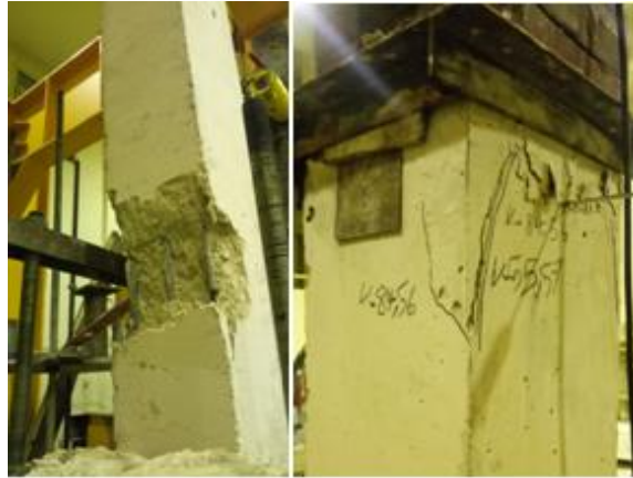
Fig. 7. The cracks of column c2 at failure under the ultimate axial load
