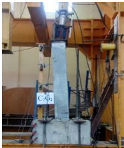
Fig. 8. The cracks of column C2G2 at failure under the ultimate axial load
