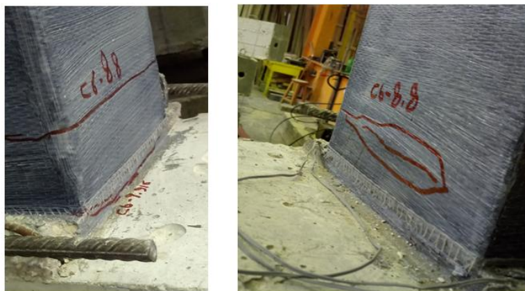
Fig. 14. The cracks of C2C2 column at failure under the lateral load. Separation of the fiber is noticed at the marked area
