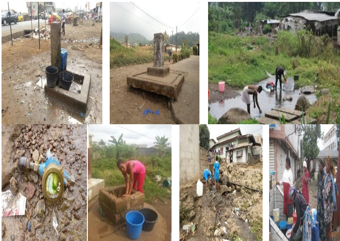
Plate 2. Nature of water supply infrastructures in Limbe
