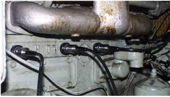
Figure 26. The installation positions of the accelerometers.
